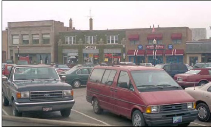
Figure B11. The Commuter Parking Lots Separates the Williams Street Train Depot from the Commercial Area
