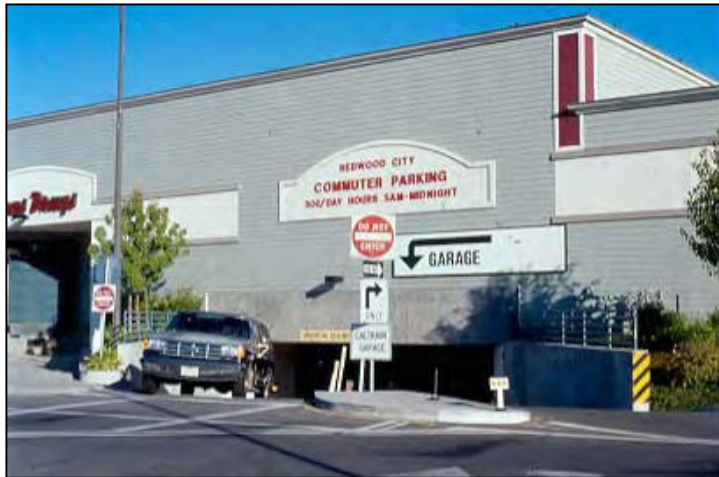
Figure 3j. Parking Facility at Station Area
