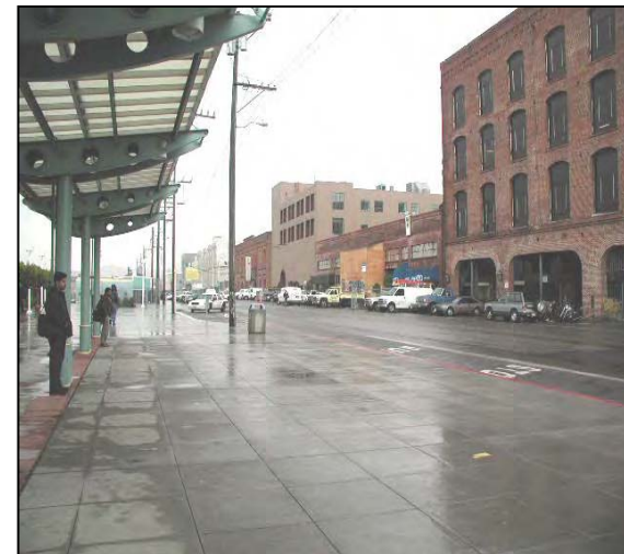
Figure B3. Renovation of Industrial Buildings to Residential Units at San Francisco Station
