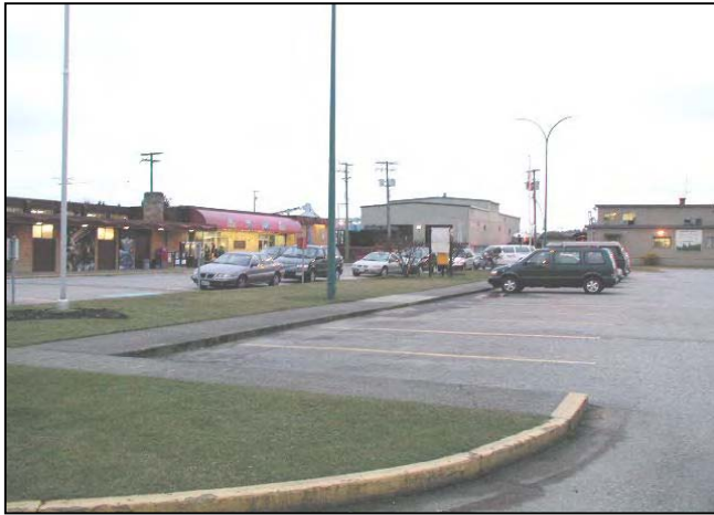
Figure B32. BC Rail Station Parking and Drop Off Facilities Near Station
